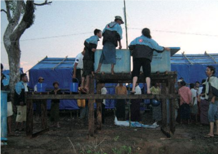
■ Setting up water tanks
