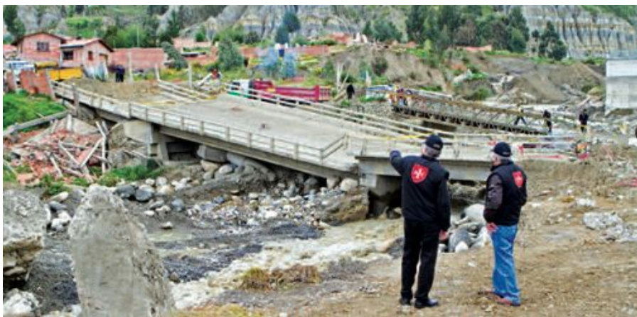
■ Inspecting flood damage in Bolivia
