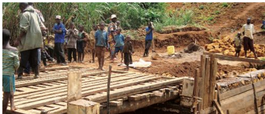
■ Keeping communications lines open: road building in DR Congo
