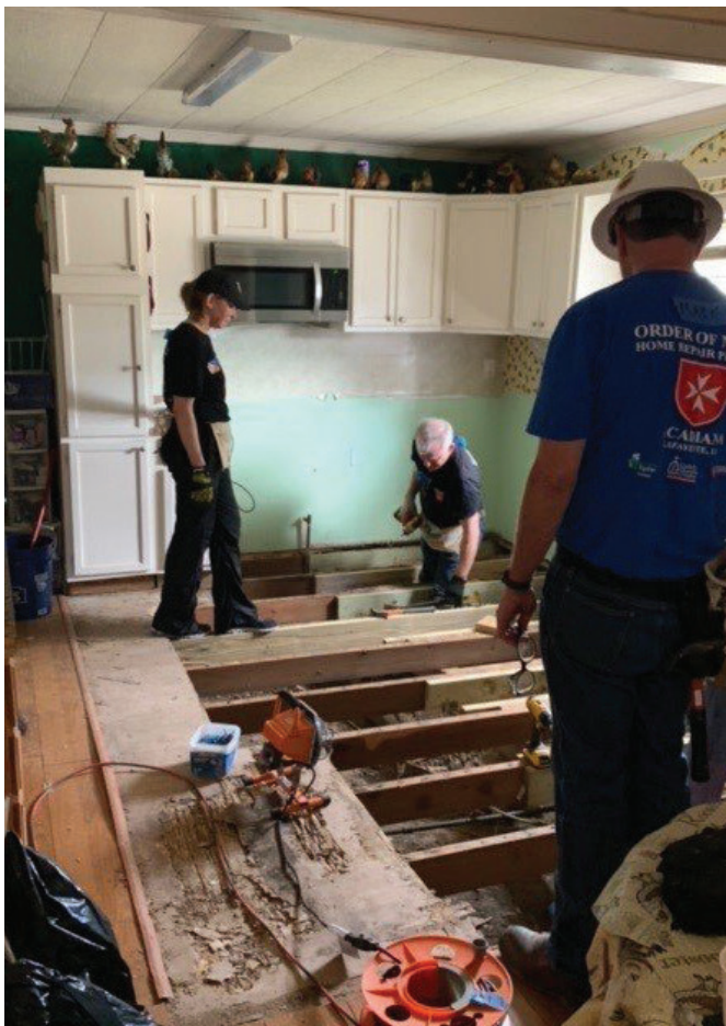
Disaster Rebuilding Program- Lafayette, LA
